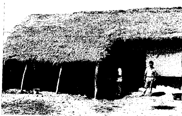
Figure 3. A shed for cattle roofed with the stems of Triticum monococcum called Chekalia
